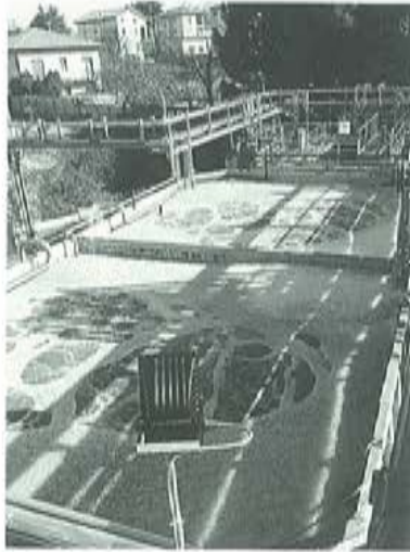
The aeration tank of the biological wastewater treatment system in Fino Mornasco.
