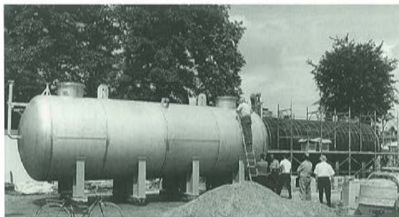
The three tanks were given a thick fireproof insulating layer.
