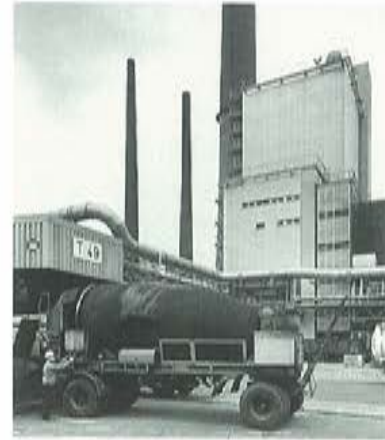
An active carbon mixer transports the liquid wastes to the Henkel power plant.
