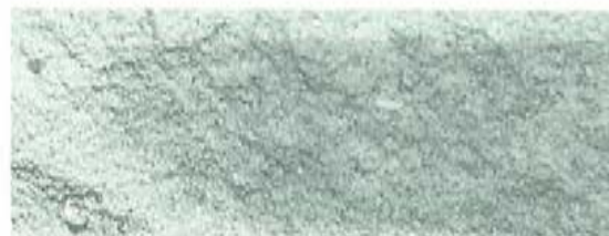
Photo above: limestone rock showing the wear of ages. Below: impregnated rock.
