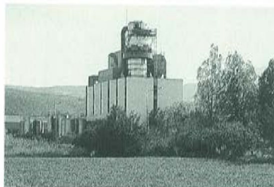
Atalanti: an end-of-stack filter ensures dust-free air.
