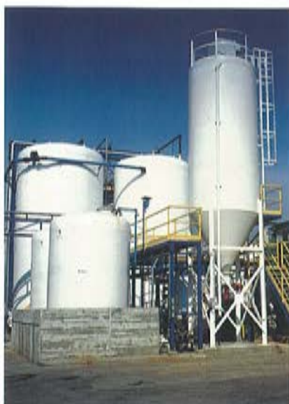
The new wastewater treatment plant in Barcelona has reduced COD loads.
