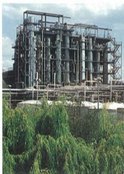
Where animal fats are handled in oleochemical production processes, as in this Düsseldorf facility, high temperatures and pressures effectively rule out any BSE hazard.
