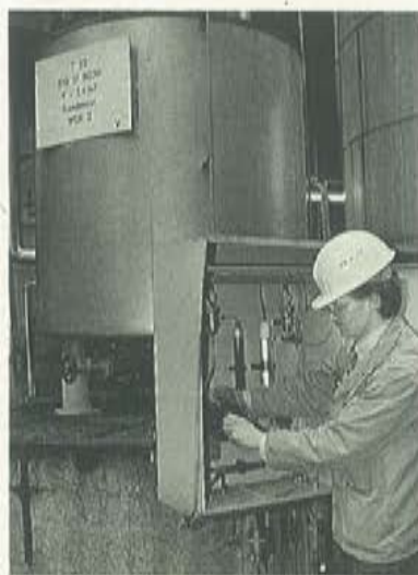
Hot condensate is collected in the tank (in the background).
