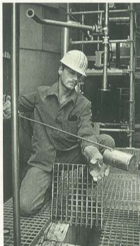
Sampling: even rainwater is analyzed, and treated if necessary, before it is allowed to flow into the plant's sewage network.
