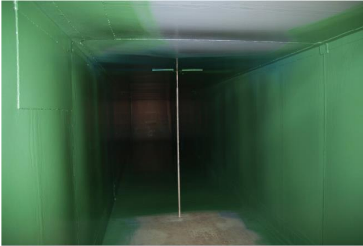
Flue gas duct after coating.
