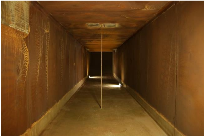
Flue gas duct of the Henkel power plant before coating in 2015.
