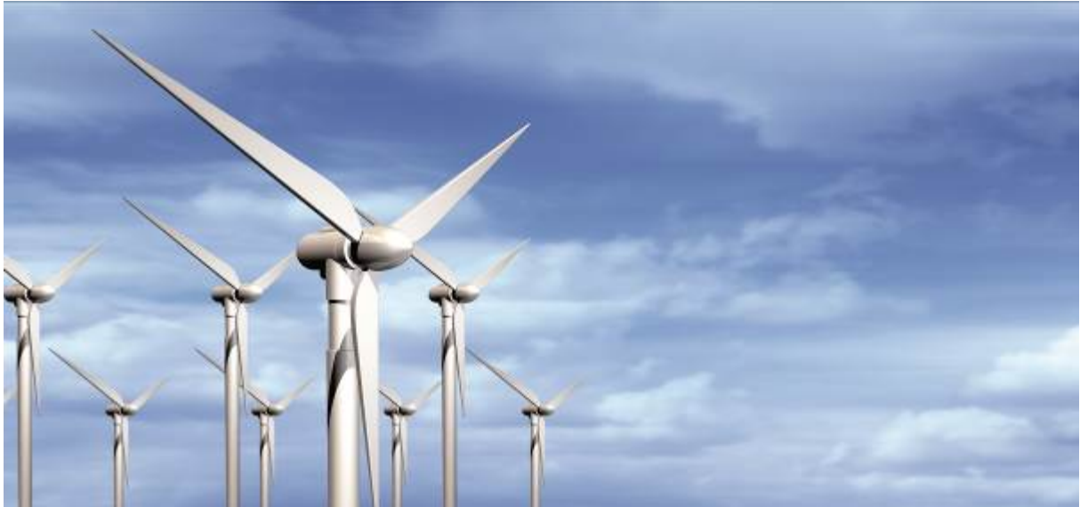
Wind turbines in operation.
