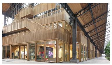
A wooden skeleton structure was constructed around the shopping, dining and event complex "Gare Maritime", using  $10,000 \text{ m}^3$  of wood. During construction, 3,858 tons of  $CO_2$  emissions were saved.
