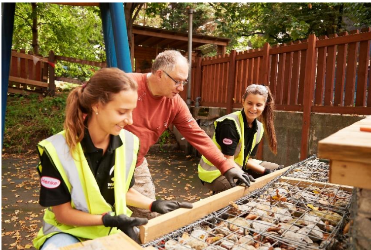
'Welcome Home' offers volunteers the opportunity to help on a personal level and to engage in dedicated construction activities. Picture: Project United Kingdom
