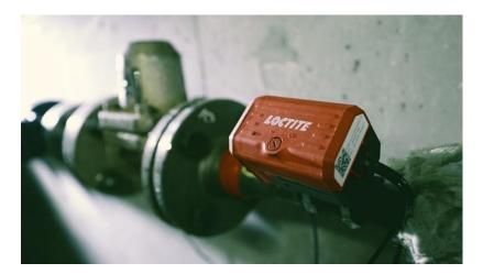
With a set of easy-to-install nano sensors applied at the inlet and outlet of the steam trap, the solution continuously gathers information about the status of the equipment.
