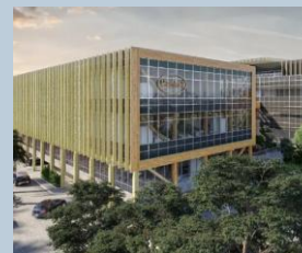
Inspiration Center in Brazil (Adhesive Technologies)
