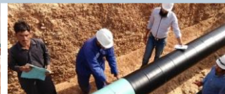
Pipeline coating & repair
