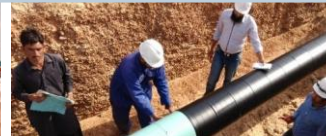
Pipeline coating & repair
