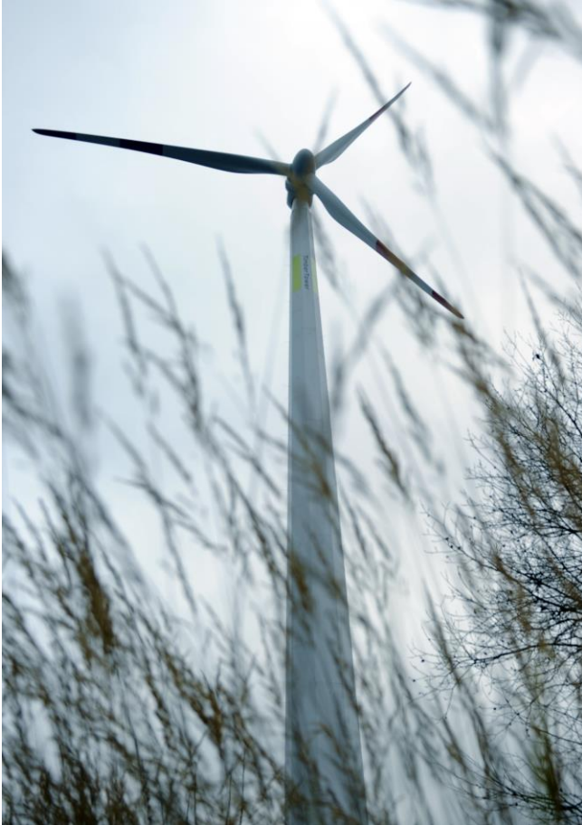
The TimberTower wind turbine mast sited in Hannover was constructed using adhesives under the Loctite (formerly: Purbond) brand.
