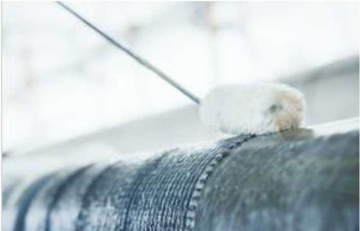
The repair system reinforces and seals steel pipes that have been designed to withstand high pressures, elevated temperatures and be highly resistant to chemicals.
