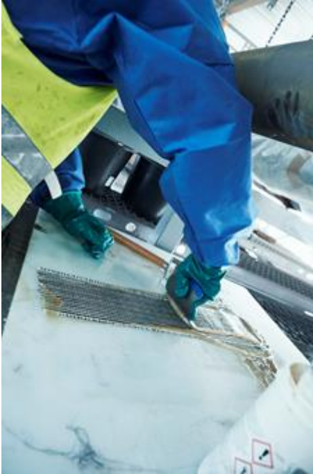
Applying LOCTITE PC 7210 to the glass-carbon fiber tape
