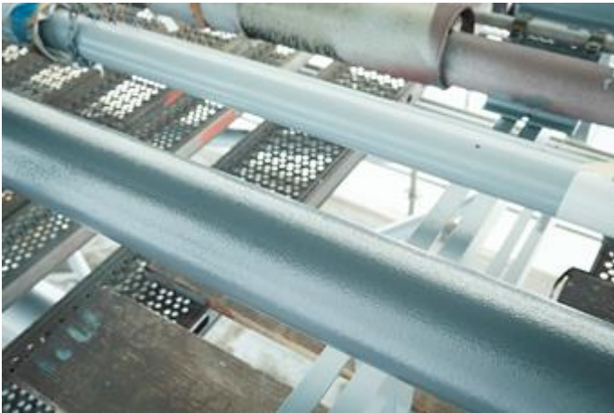
A steel pipe after coating with LOCTITE PC 7255 sprayable ceramic topcoat as the protective finishing layer
