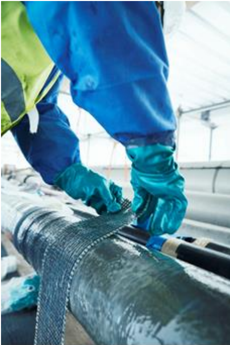
The repair system reinforces and seals steel pipes that have been designed to withstand high pressures, elevated temperatures and be highly resistant to chemicals.
