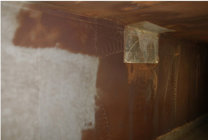
Sulfuric acid corrodes steel
