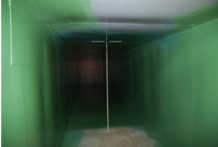
The flue gas duct during application work
