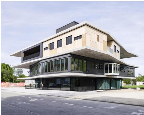
In May 2016, the research and accommodation building NEST (Next Evolution in Sustainable Building Technologies) was inaugurated at EMPA Dübendorf/Switzerland. Here for the first time, cross-laminated beech timber elements were bonded with the Loctite Purbond primer system to create the load-bearing structure. (Photo: Roman Keller)
