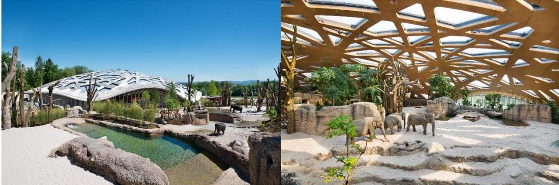
The canopy-like freestanding domed roof of the elephant house, which opened at Zurich Zoo in Switzerland in mid-2014, consists of high-load cross-laminated timber elements bonded with an adhesive of the Loctite HB S Purbond line. With this fiber-free adhesive facilitating a production process which is as individual as it is reliable, it was possible to meet the high demands on structural strength and shape stability in the laminated panels employed. (Photos: Jean-Luc Grossmann)
