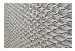
The 3D Printed wall in the Henkel Innovation and Interaction Centre, made from Loctite products and designed by Jennings Design Studio, Dublin and Aectual, Netherlands.
